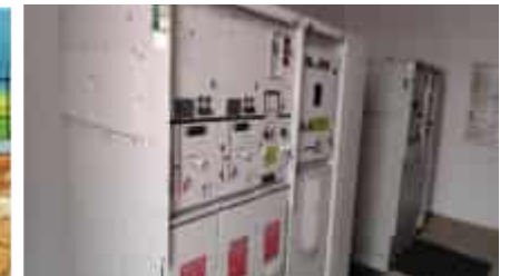
Dedicated RMU for each plot for 33/11 Electricity and Optical Fiber connection
